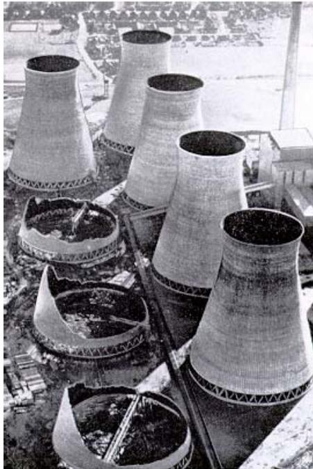
Figure 3: Collapsed cooling towers in Ferrybridge C power plant. On 1 November 1965, the wind of 85 mph was blowing from the right to the left side of the photo.
