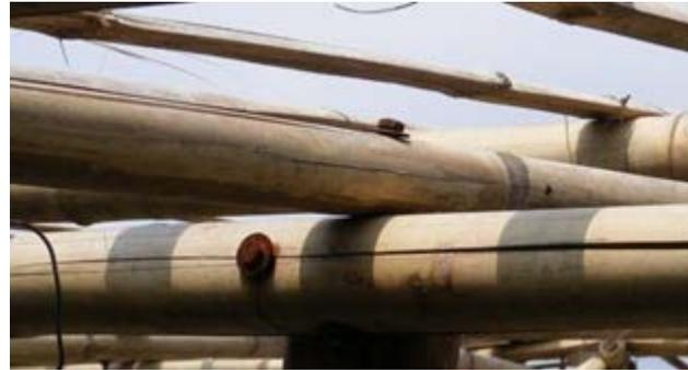
(b) Splitting at bolted connections
