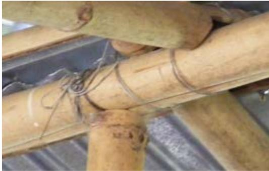
(a) Beam splitting at joint
