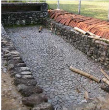
a) stone submerging pool for treating with a solution of water and Octabor
