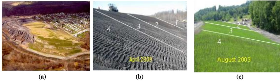
Figure 1.1 Coal refuse pile in the Mather site: (a) original condition with barren lands, (b) with the top 61 cm surface pile just reclaimed, and (c) three months after the reclamation with BR. (These photographs were taken by Alcoa Inc.)
