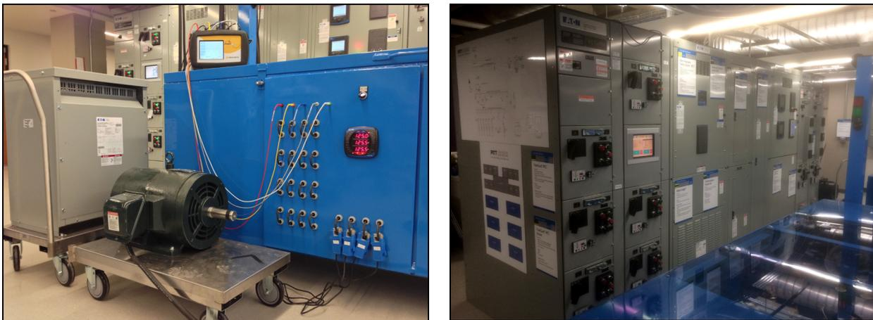
**Figure 8.1: Portable Motor Units (Left) and Motor Control Center (Right)**
