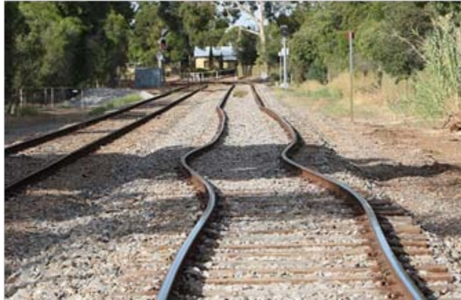
Figure 1.2. Thermal buckling in a continuous welded rail (Robertson, 2012).
