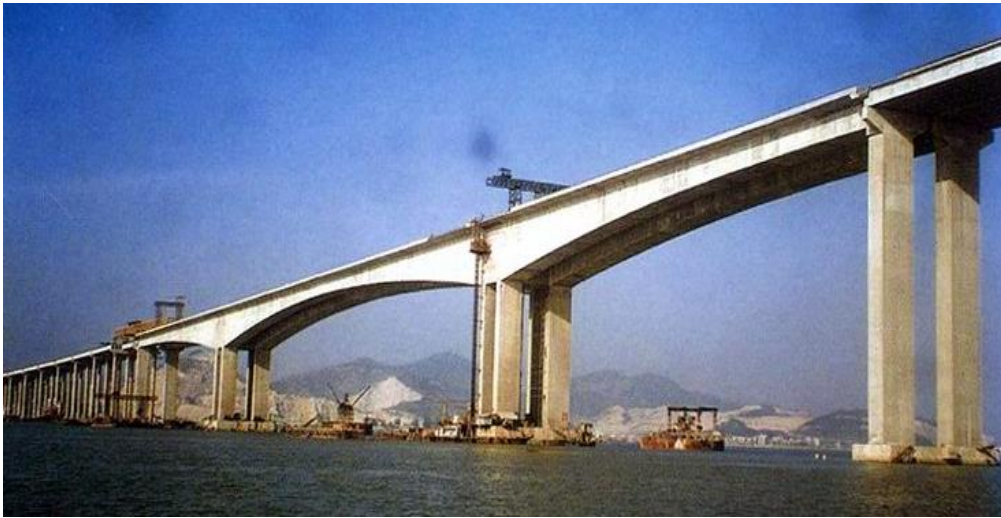
Figure 6. Humen Bridge Auxiliary Channel Bridge
