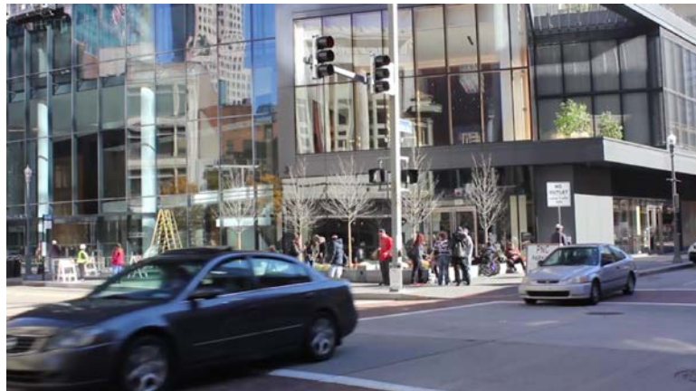
Figure 11: PNC Tower: Street View
