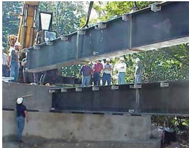
b) Use as bridge girder (VA Route 601 over Dickey Creek)
