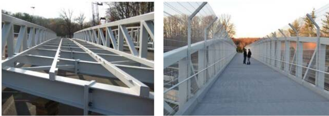
Figure 1.4 Pedestrian bridge fabricated of pGFRP members (Composite Advantage 2015)
