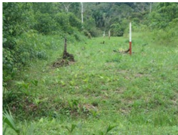
Figure 62: Poles behind Cesar's house demarcate the subterranean tube that transports crude oil.
