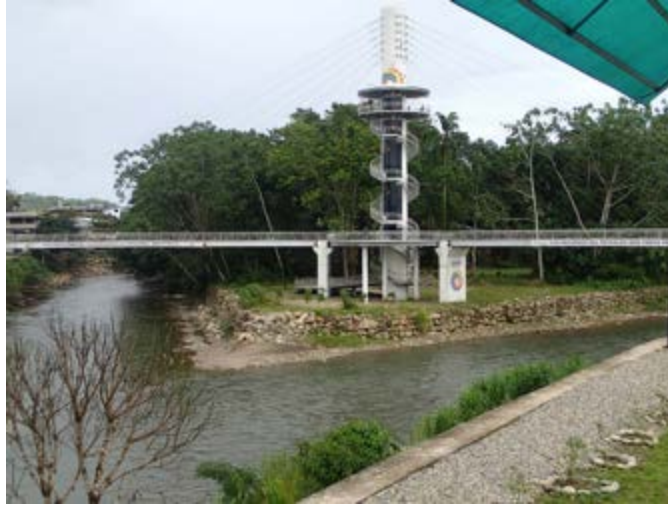
Figure 64: New bridge in Tena.
