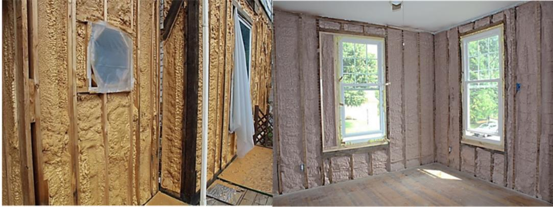
**Figure 18: SPF application first floor exterior façade (left) and second floor interior wall (right)**
