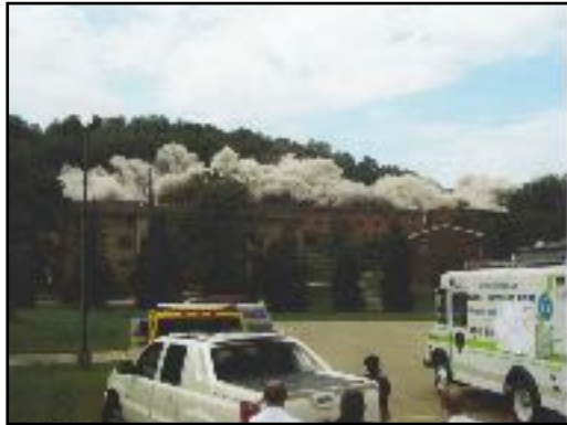
Figure 19. Sequence showing demolition of the Garfield Heights Towers in 2005. Source: Housing Authority of the City of Pittsburgh.
