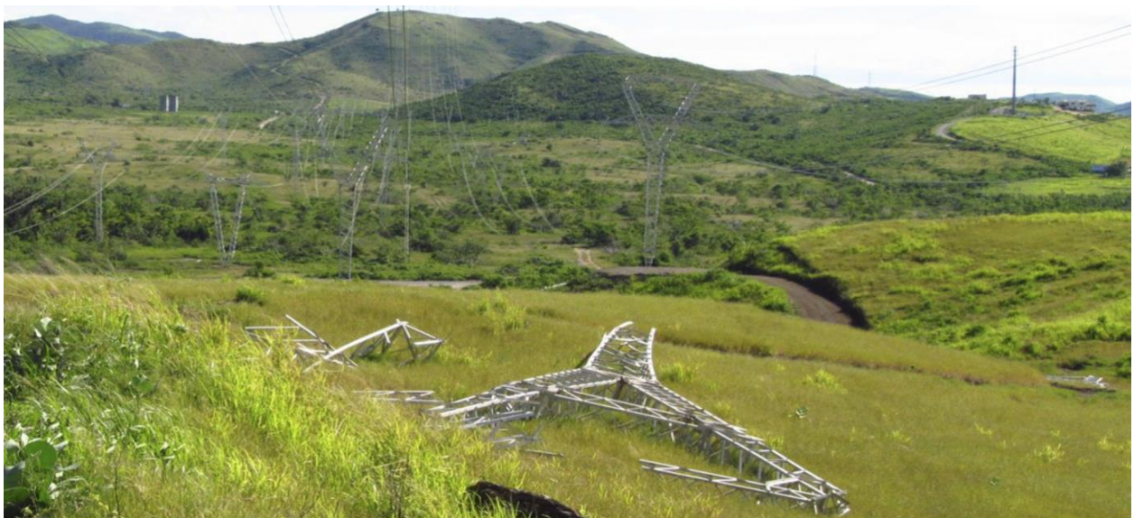
Figure 3. Damage to high voltage towers in the Southern part of Puerto Rico. (© Alexis Kwasinski, used with permission)
