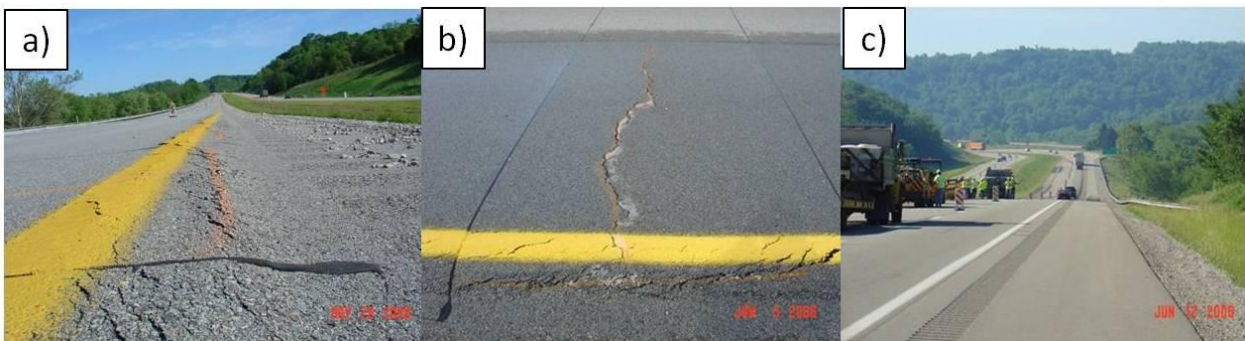
Figure IV-23 – Panel LW-54 photographs showing (a) lane-to-shoulder drop-off, (b) transverse and longitudinal cracking between saw cuts, and (c) final subsidence basin (Photographs from PA DEP files).
