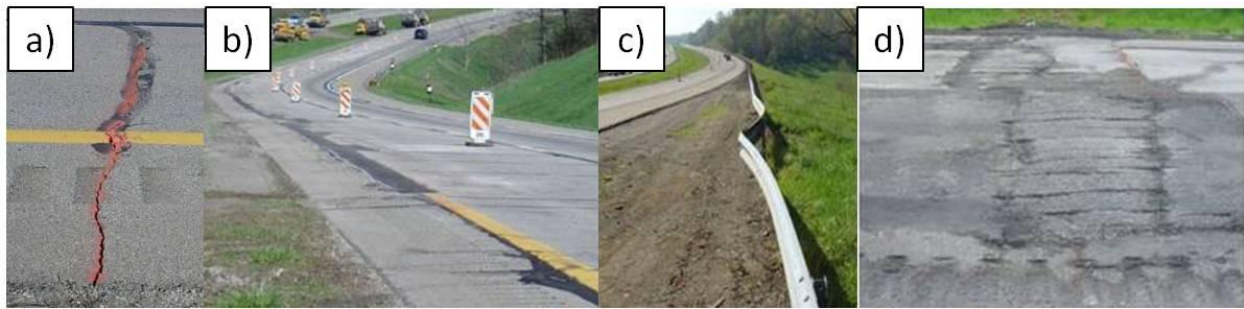
Figure IV-20 – Panel LW-51 photographs showing (a) spalling of transverse joint, (b) lane-to-shoulder separation, (c) compression of guard rail, and (d) blowup (Photographs from PA DEP files).
