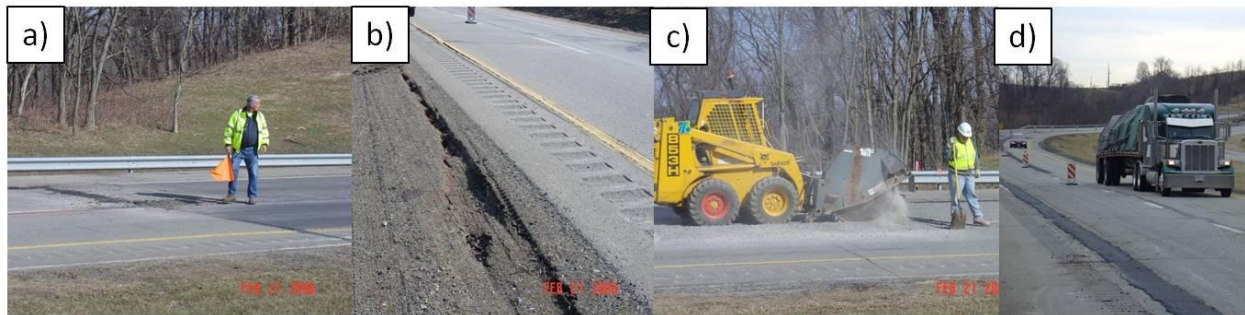
Figure IV-13 – Panel B3 photographs showing (a) a transverse compression heave, (b) lane-to-shoulder separation, (c) blowup compression bump being milled, (d) single lane restrictions with longitudinal patching, February 21, 2006 (Photographs from PA DEP files).
