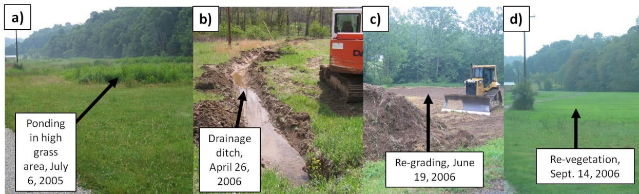
Figure VII-11 – Photographs of a commonly used method to repair settlement impacts after ponding resulted within a field or pasture (Photographs from PA DEP files).
