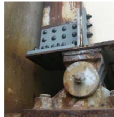
b) bolted repair of web-flange region and bearing stiffener (Wakabayashi et al. 2013)
