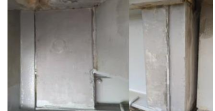
a) I-91 bridge over rail corridor b) PVC distribution of UHPC c) completed repair Figure 12 Field Implementation of UHPC Repair Reported by Hain and Zaghi (2021)
