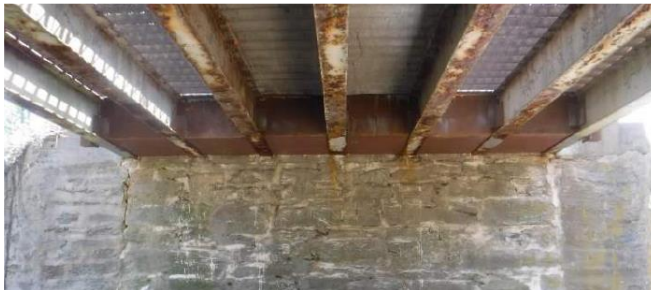
c) steel-formed concrete encasement at abutment of bridge having embedded beams (Bridge I)
