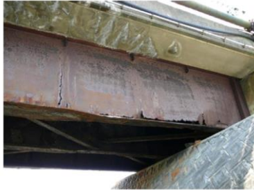
Web failure, Korea (Ahn et al. 2013)
