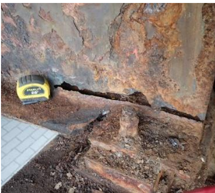
a) Pattern M1 damage (b = 17 in.; a = 1.5 in.)
