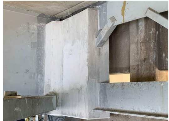
b) completed repair of diaphragm
