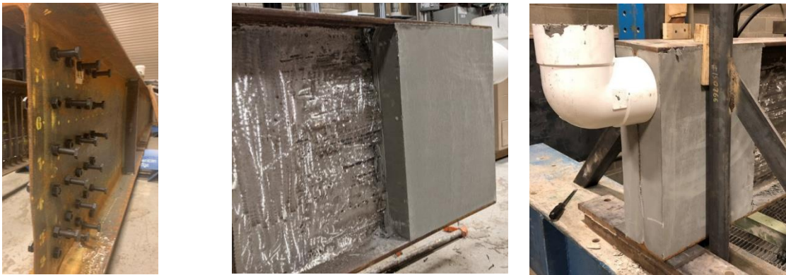
Figure 35 UHPC Repair Detail for Girder 4
