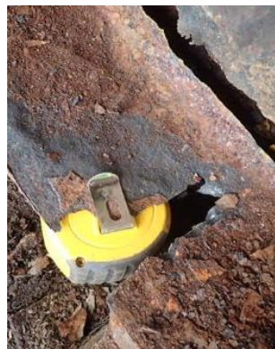
b) apparent cut through bottom flange
