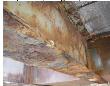
c) steel-formed concrete encasement at abutment of bridge having embedded beams (Bridge I)
