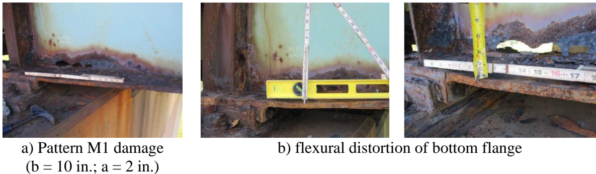
Figure 23 Flexural Distortion of Flange Accompanying Significant Pattern M1 Damage (Bridge J)
