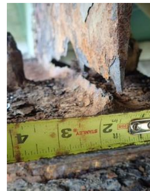
c) lateral distortion of web
