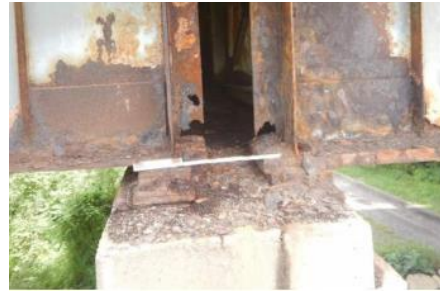
b) Welded patch web plates above bearings at spans 3 and 4 over pier 3 (Bridge D)
