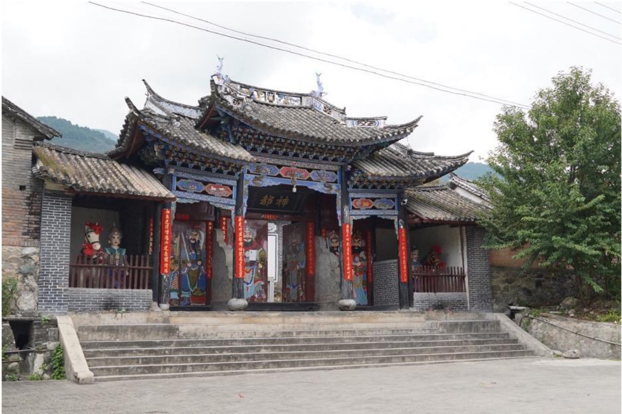
Figure 5 The exterior of the Shendu temple. Photograph by author, October 13, 2020.
