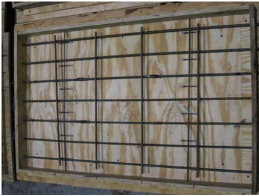
(a) Typical Formwork
