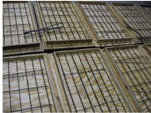
(b) Slab forms prior to casting
