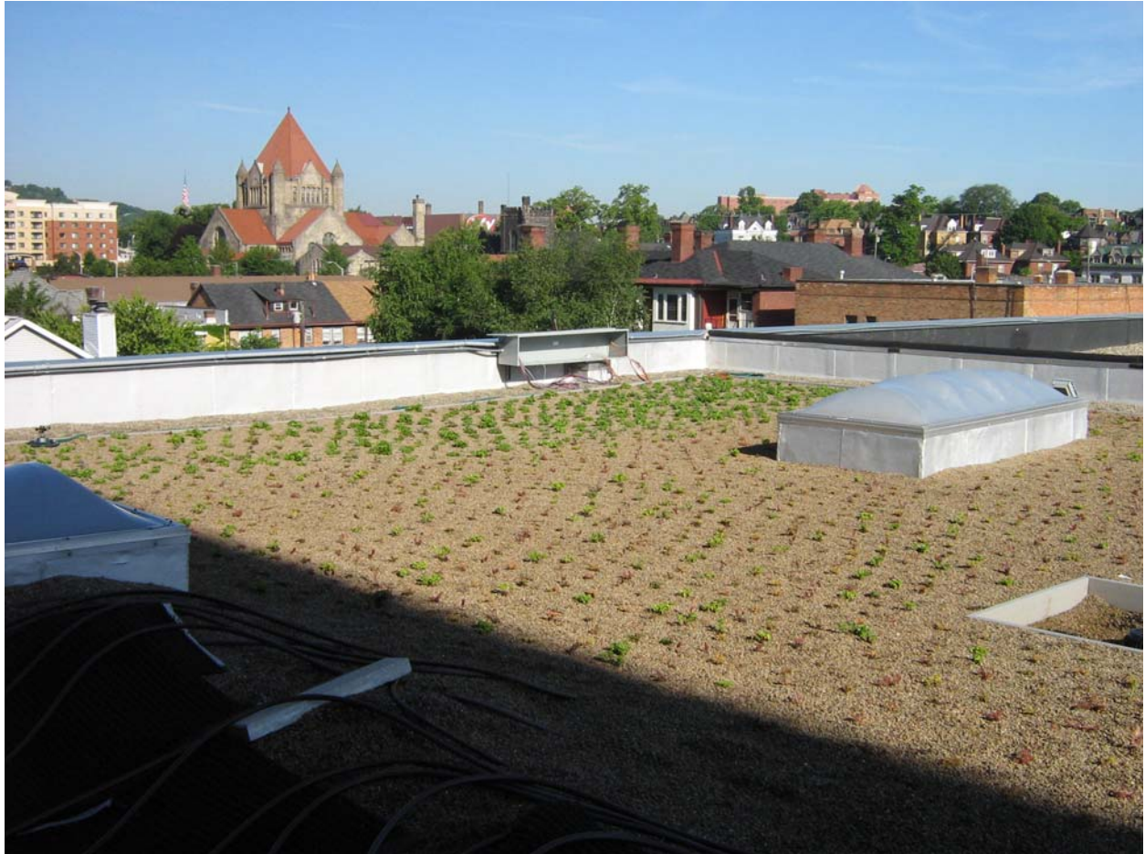
Figure 8 - Giant Eagle Green Roof Just After Installation of Plants
