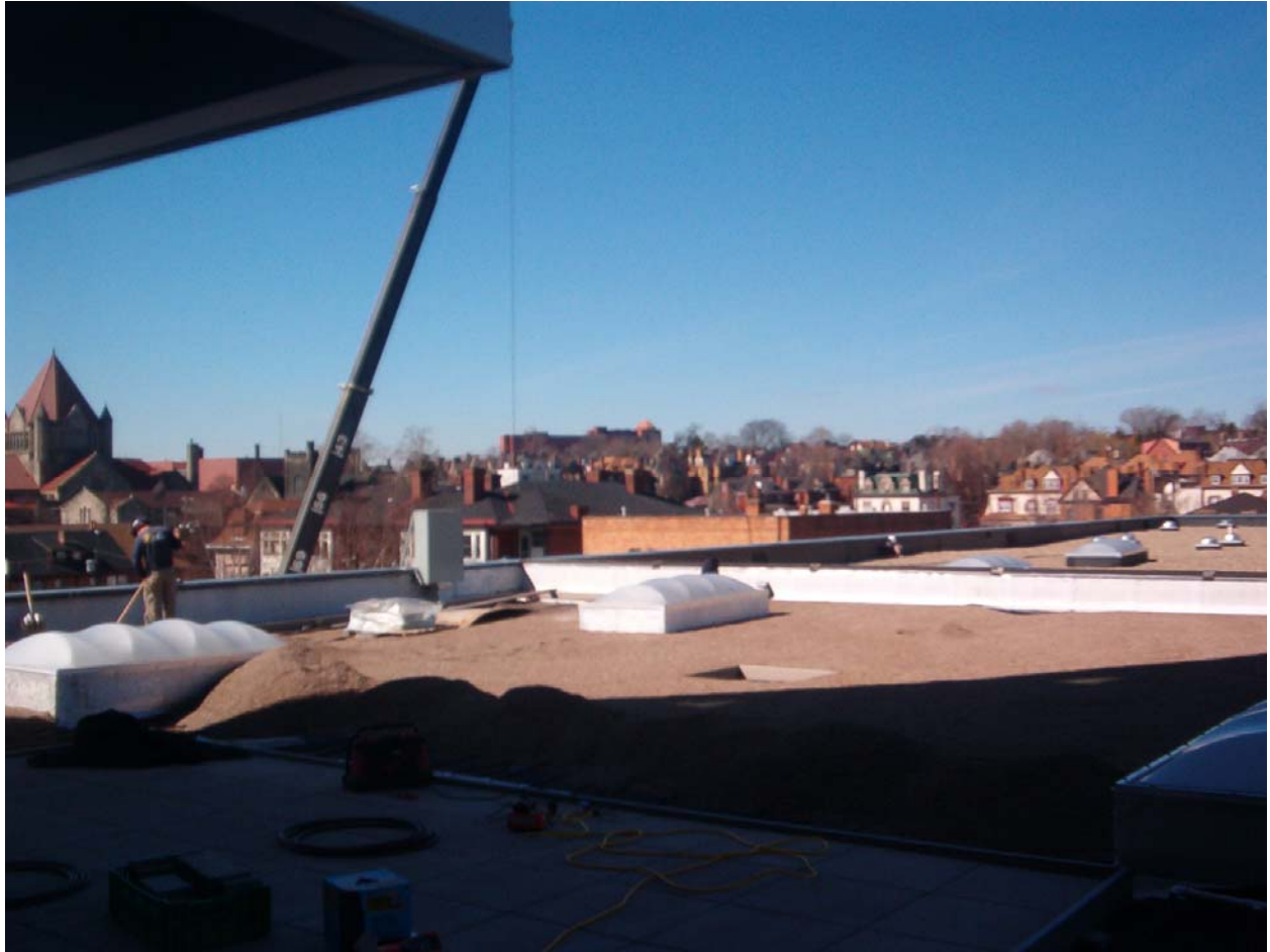
Figure 7 - Giant Eagle Green Roof as Soil is Installed
