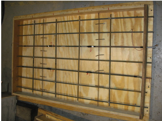
(a) typical formwork
