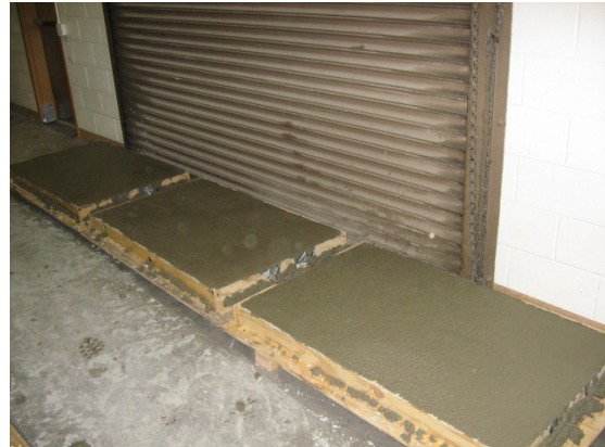
(b) three slabs after casting
