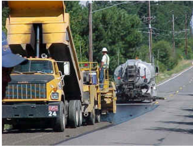
Figure 4. Application of slurry seal before placing chips ( www.cityofsalem.net )
