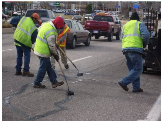
Figure 1. Crack sealing being performed ( www.chipseal.com )
