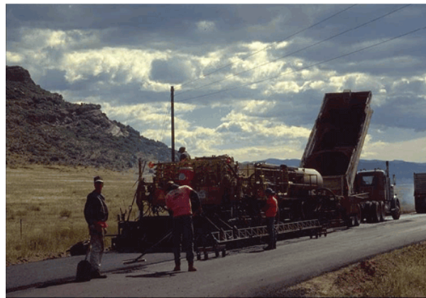
Figure 6. Heat Scarification in progress ( www.fhwa.dot.gov/pavement/recycling/98042/09.cfm )
