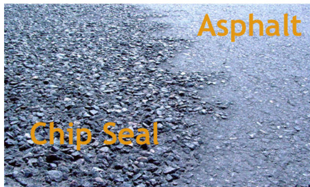
Figure 2. Chip Seal ( www.chipseal.com )
