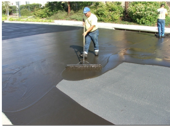
Figure 3. Slurry Seal being laid on the pavement surface ( www.unitedpavinginc.com/services.php )
