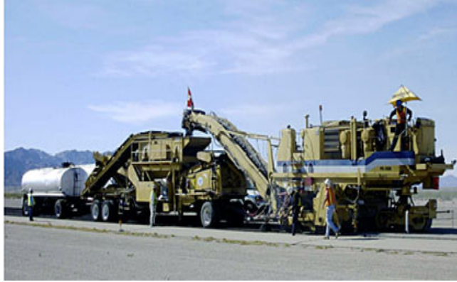
Figure 11. Cold In-place Recycling ( www.fhwa.gov )
