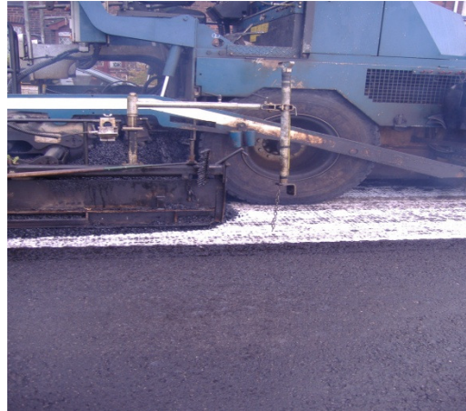
Figure 9. Microsurfacing layer ( www.fhwa.gov )
