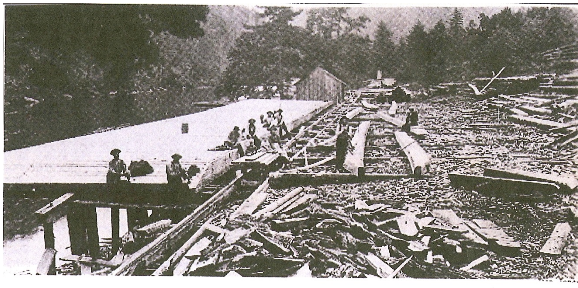
Figure 6.1. Log raft under construction on the Clarion River south of Portland Mills in Elk County. Log rafts were constructed upside down and then flipped right-side up into the river. 138
