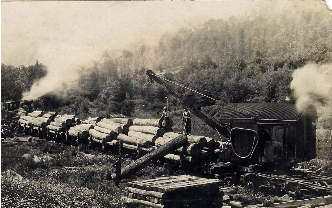
Figure 5.7. Hall and Kaul's Barnhart steam-operated loader, essential to the efficient loading of logs onto railroad cars. This machine is considered by some to be nearly as important to logging as the Shay locomotive. 112
