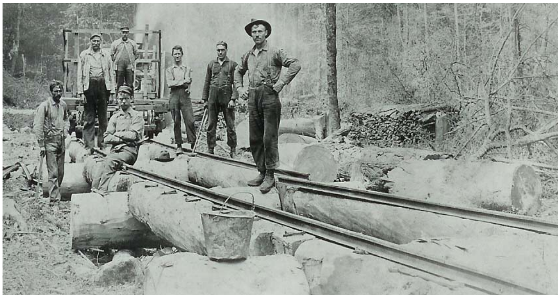
Figure 4.7. Logs laid parallel to the rail provided temporary beds for logging railroads. 77
