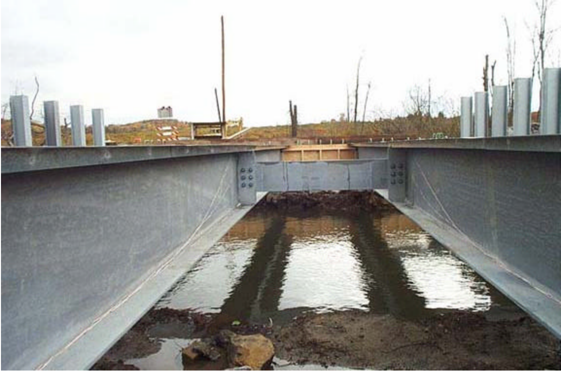
Figure D-8 - Boyer Bridge, Diaphragm
