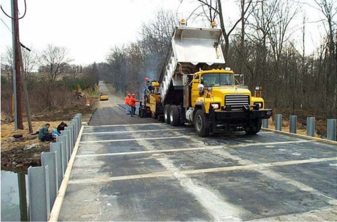
Figure D-11 - Paving over the FRP deck, Boyer Bridge
