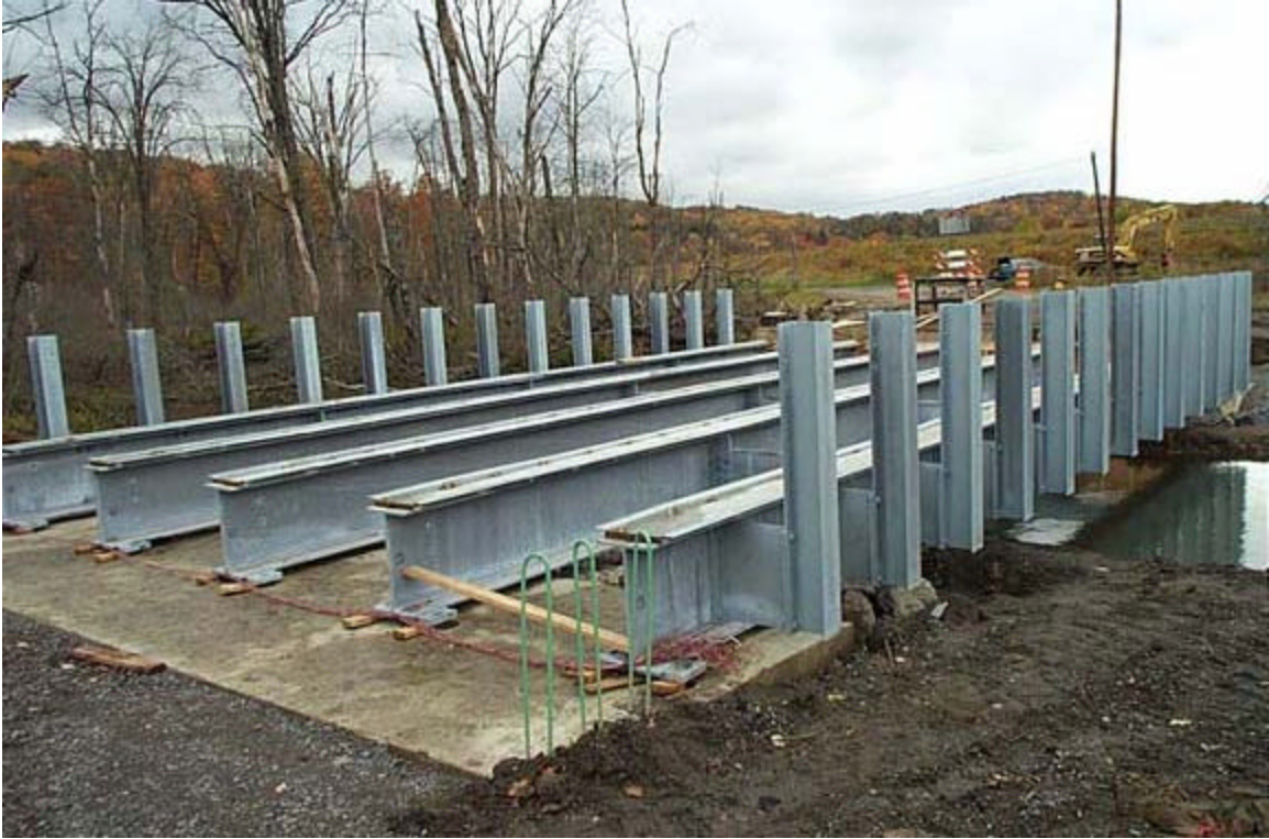
Figure D-17 - Strain gage lead wires gathered at forward abutment
