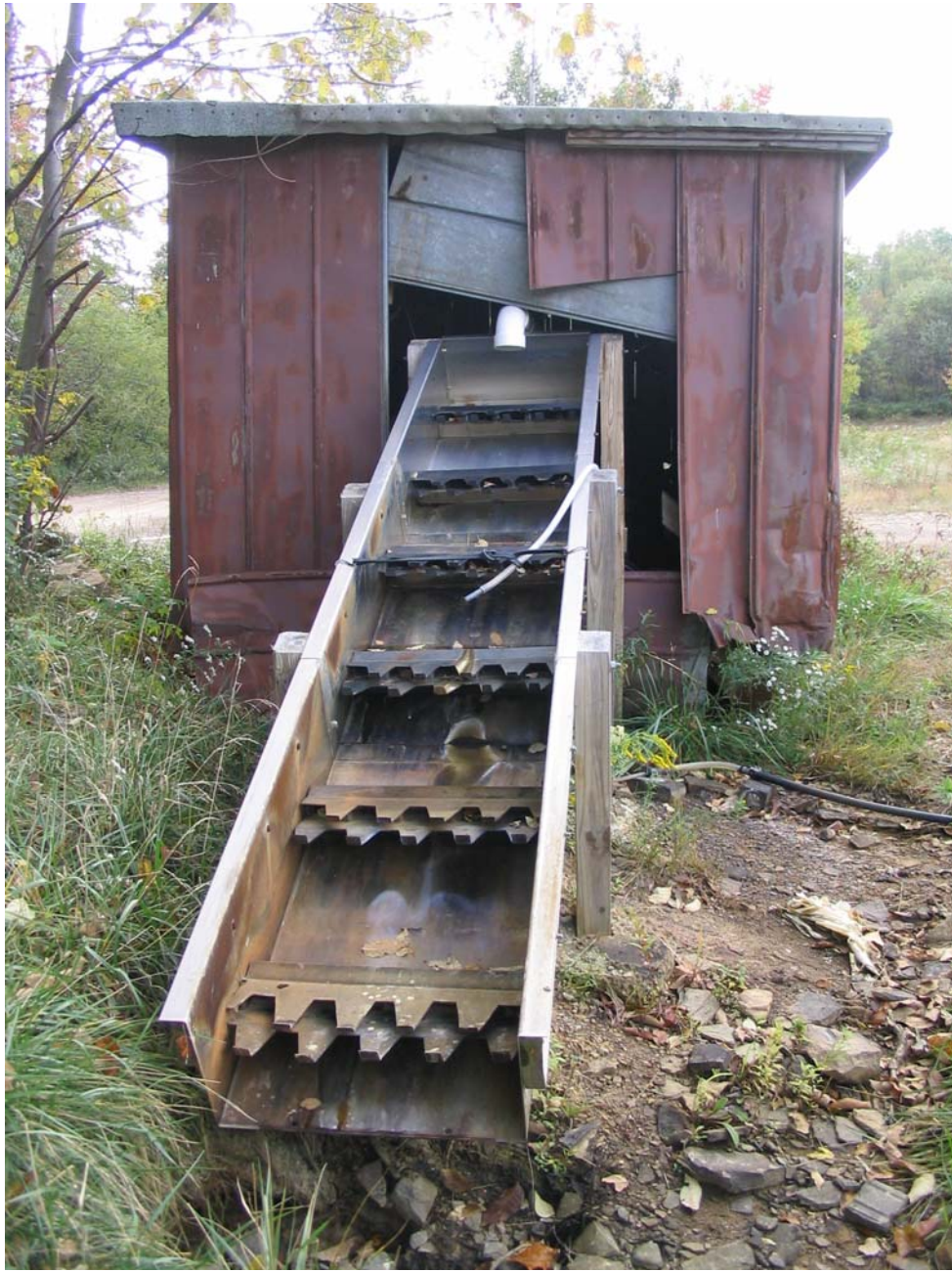
Figure 22. The water enters from the top through the PVC pipe and continues down the trough where caustic soda is added and mixes with the water
