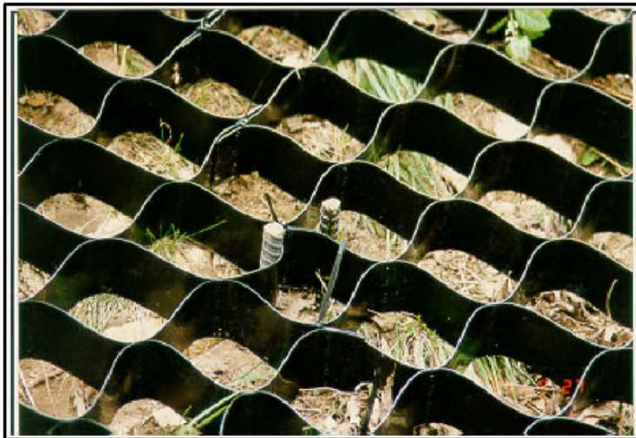
GEOWEB COVER SYSTEM PLACED ON STEEP SLOPE CONDITION
