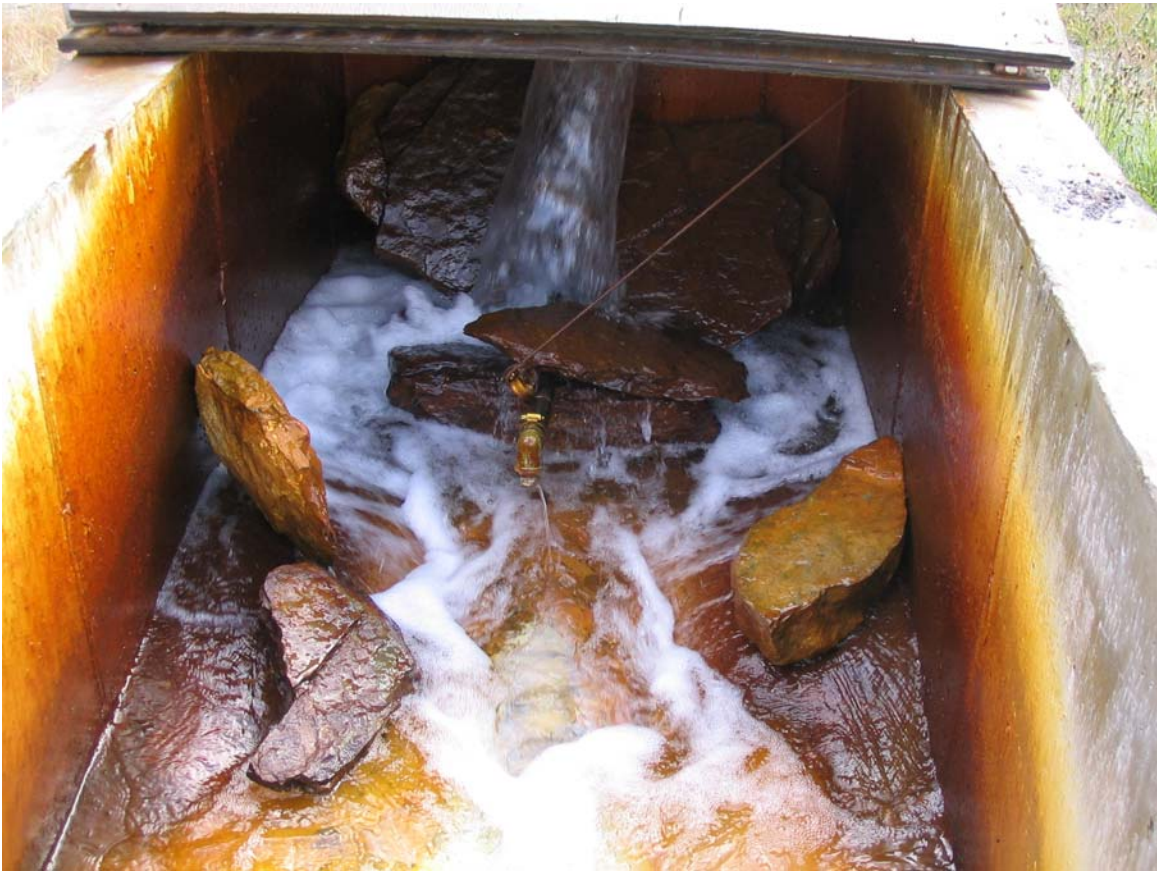
Figure 19. Mixing technique found at a chemical treatment system for acid mine drainage in central Pennsylvania. A cement box filled with large rocks allows for turbulent mixing of water and caustic soda
