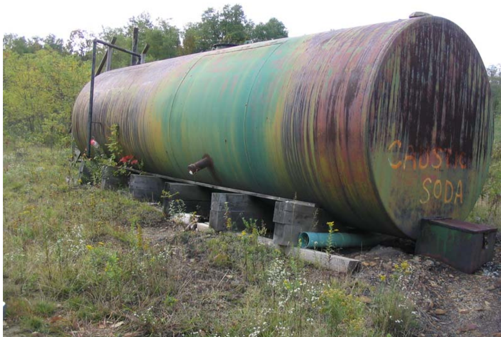
Figure 1. A 10,000 gallon tank holding sodium hydroxide
