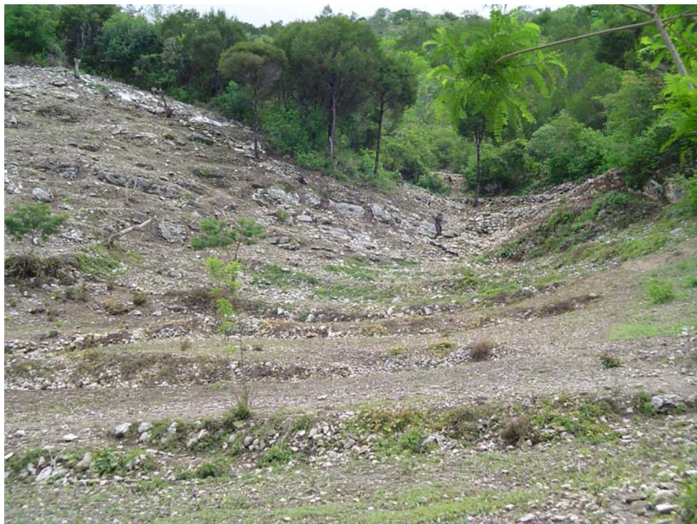
Figure 4-13 Check Dams in the Background and Dryslope Terraces in the Foreground at MR 52
