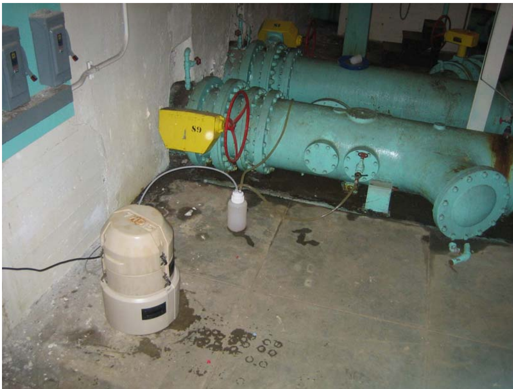
Figure 16. Herron Hill Pump Sta. (A10) - Autosampler connection to pressure main.
