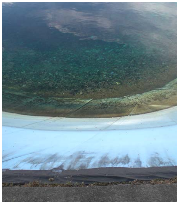
Figure 29. Sediment accumulation in the southeast corner of the east Highland No. 1 Basin.
