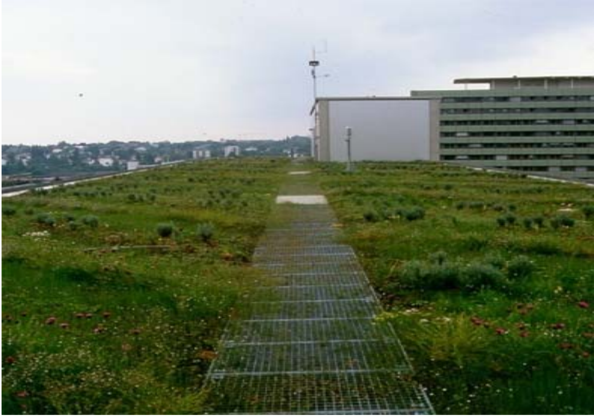
Figure 2. Typical extensive green roof (Soka-Bau green roof case study 2009)
