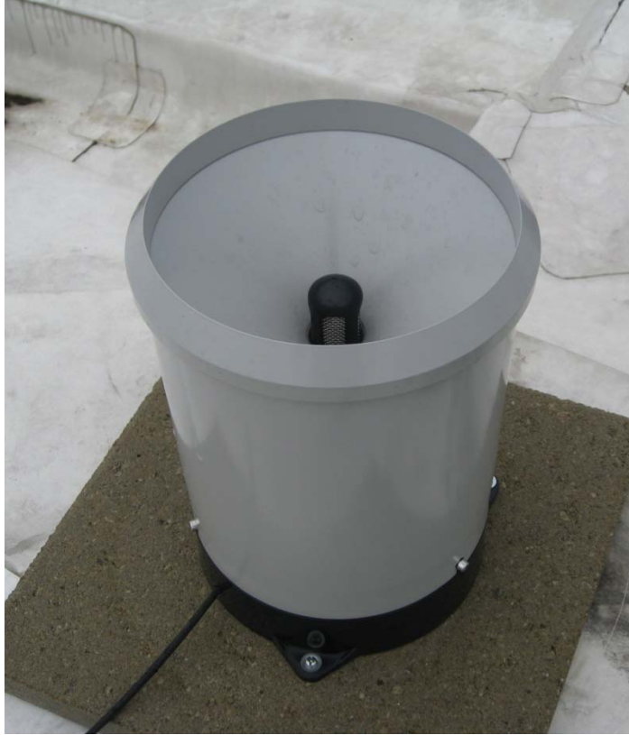
Figure 17. Rain gauge installed on the roof
