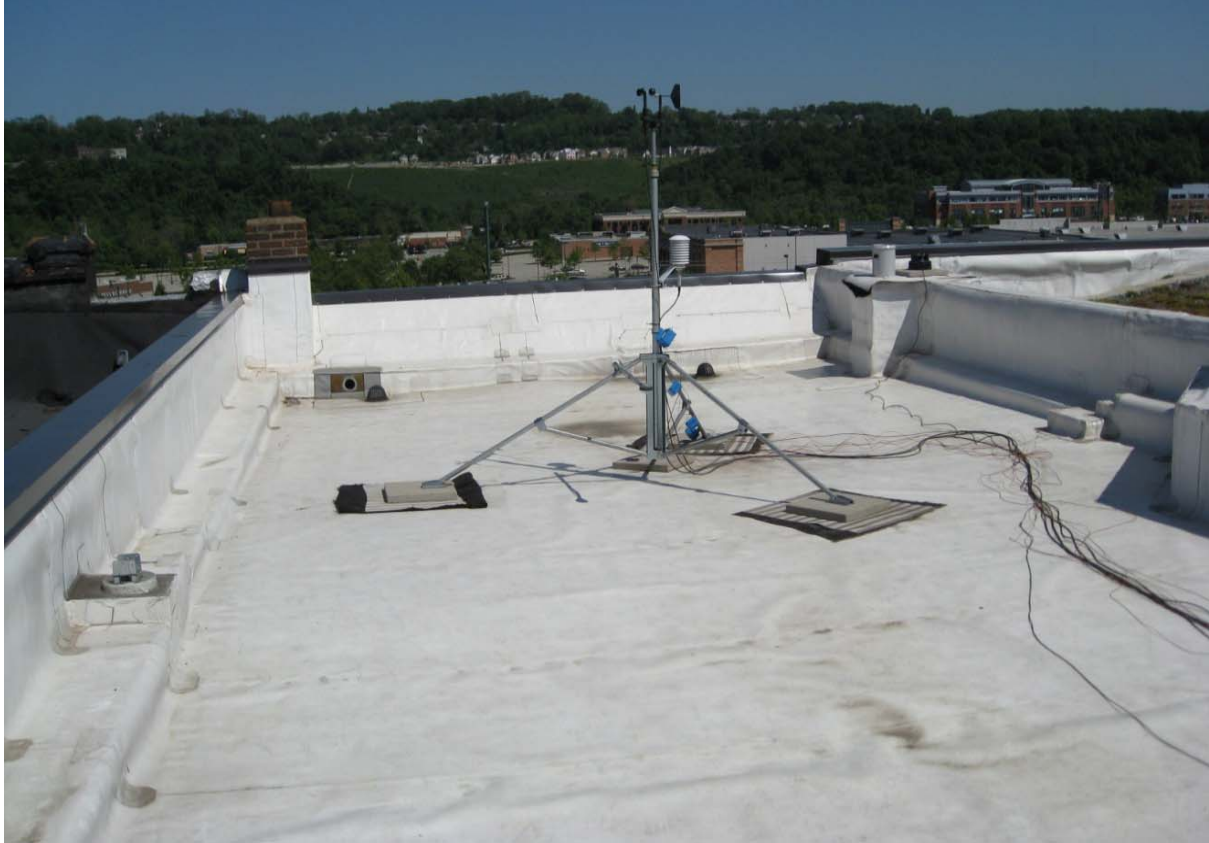
Figure 15. Control roof at Homestead site
