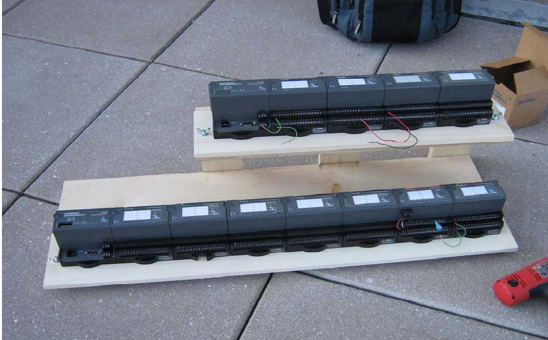
Figure 25. National Instrument Fieldpoint Dataloggers at Giant Eagle site (Bliss, 2007)
