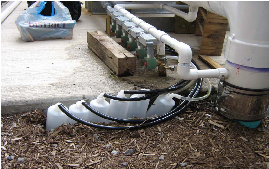
Figure 21. Solenoid Valves and Sample bottles at Giant Eagle site (Bliss 2007)
