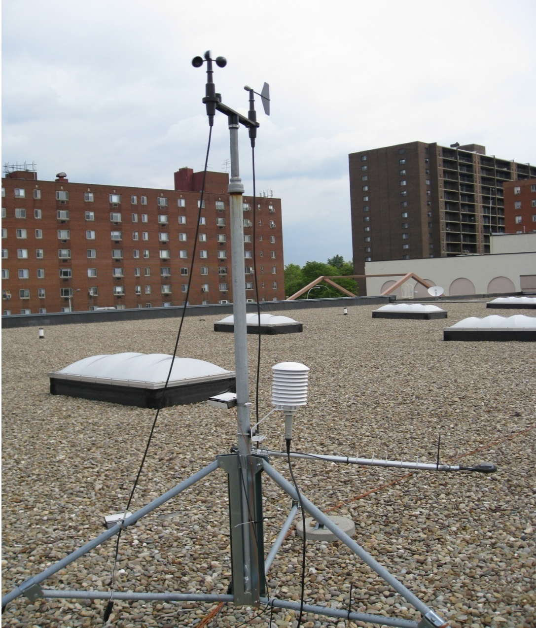
Figure 9. One of the Tripods for monitoring temperature at control roof side (Giant Eagle)
