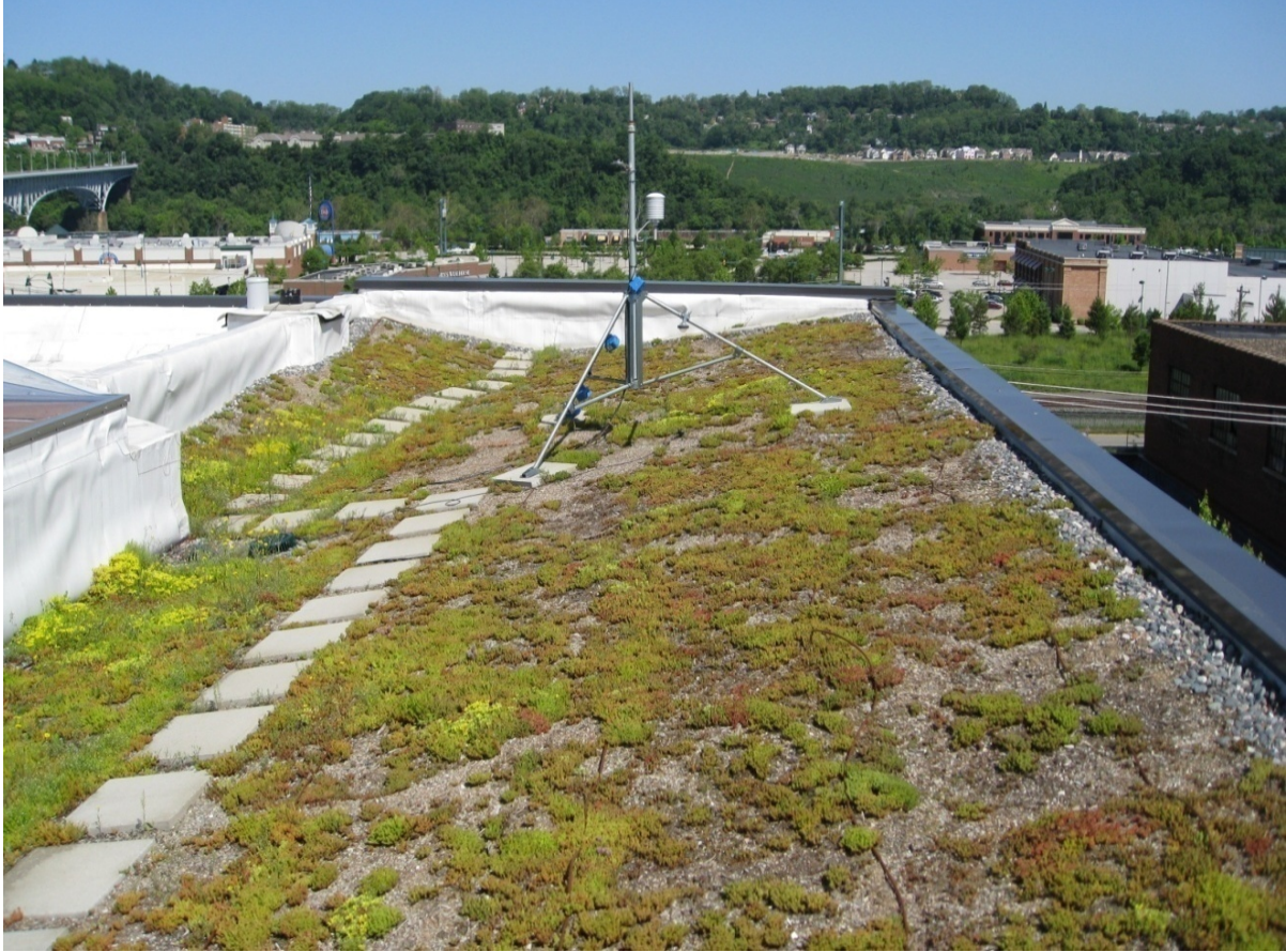
Figure 14. GLT Green roof at Homestead site
