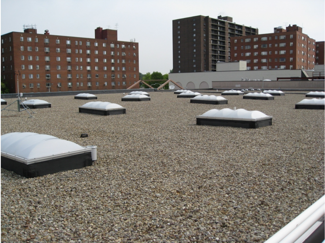
Figure 7. Control roof on the top of the Shadyside Giant Eagle supermarket
