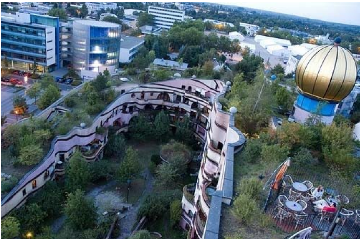
Figure 1. An intensive green roof on the top of Waldspirale, a residential building complex in Darmstadt, Germany
