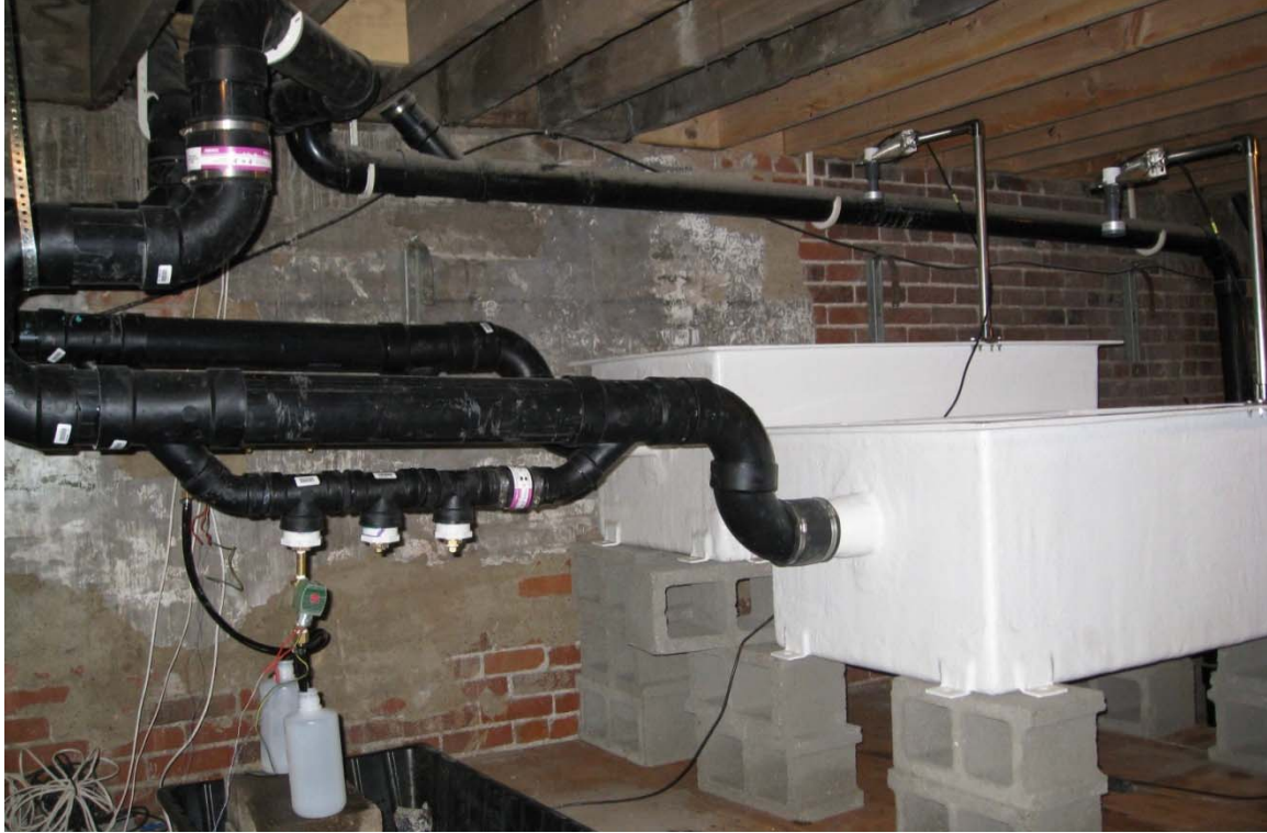
Figure 16. Drainage system at Homestead Site
