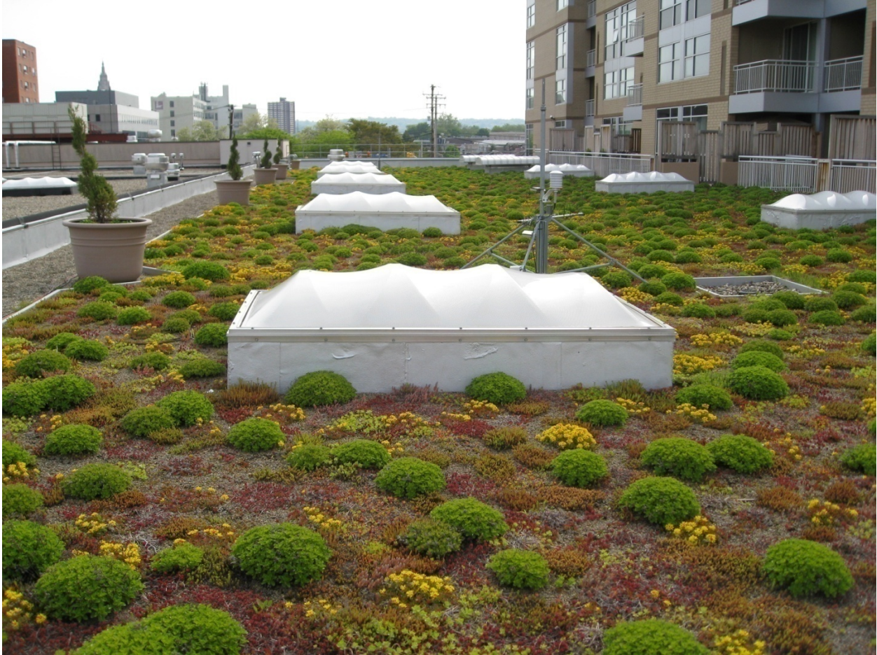
Figure 6. Green roof on the top of the Shadyside Giant Eagle supermarket
