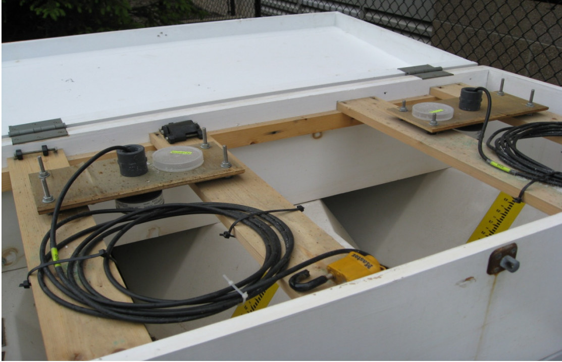
Figure 19. Ultrasonic sensors installed at Giant Eagle site
