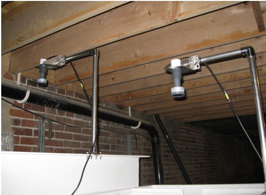
Figure 20. Ultrasonic sensor installed at Homestead site
