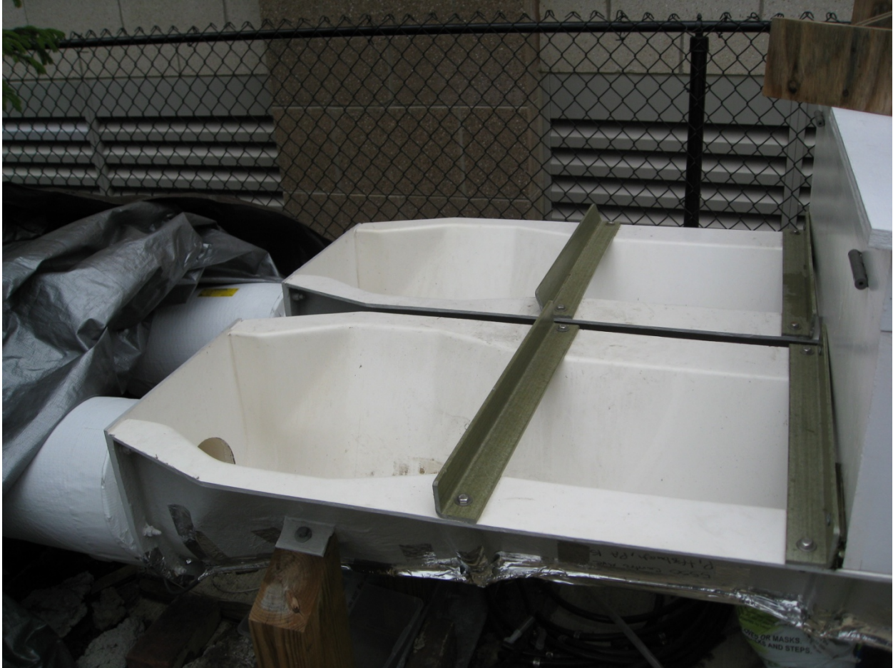
Figure 10. Flumes for runoff drainage at Giant Eagle site
