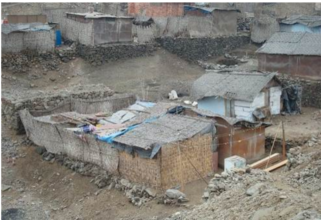
Figure 125. Perishable quadrangular structures from a modern urban shanty town of Lima. Roofs and walls are made of reed mats. Notice the low stone wall in the nearest hut and the stone platforms in the others.
