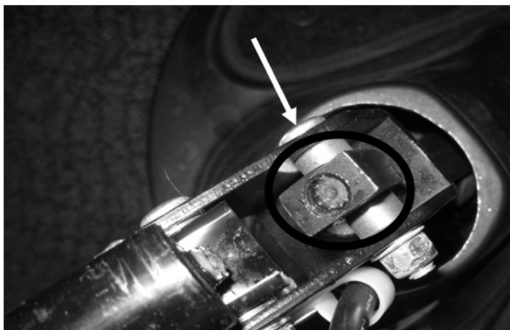
Figure 7. Close view of failure in tiller pivot. The bolt holding the adjustment strut to the tiller assembly snapped.
