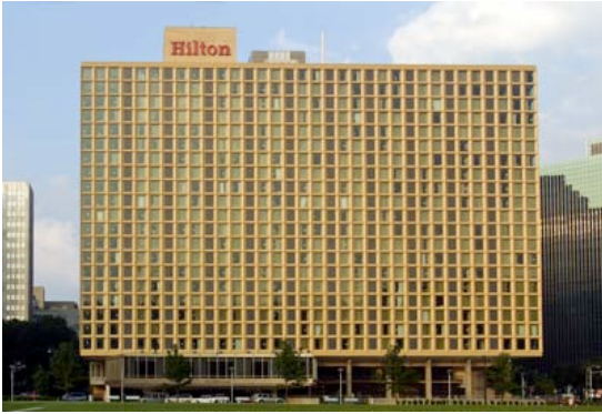
(a) Pittsburgh Hilton and Towers (Glass, Steel, and Stone)
