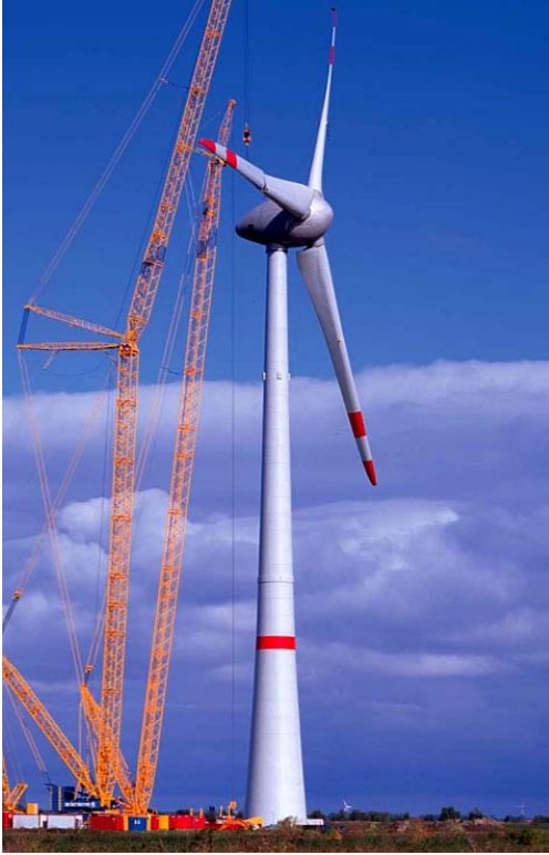
(a) World's largest HAWT, the Enercon E-126. Power capacity of 6 MW, can produce 20 million kWh of electricity, enough to power almost 1800 average US homes per year. Rotor blades are 126 m long. (photo: newlaunches.com)
