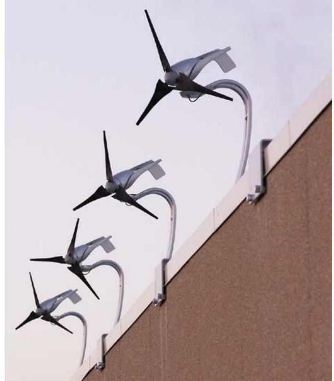
(b) Aerovironment's AVX1000 small-scale wind turbine mounted along a parapet at Kettle Foods manufacturing facility in Beloit, Wisconsin. 18 turbines projected to generate 28,000 kWh/year. (Photo: renewableenergyworld.com).
