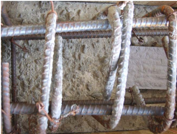
(a) Typical interface surface; Concrete Repair Institute standard surface profile chip #9 (CSP9) shown at right of image.
