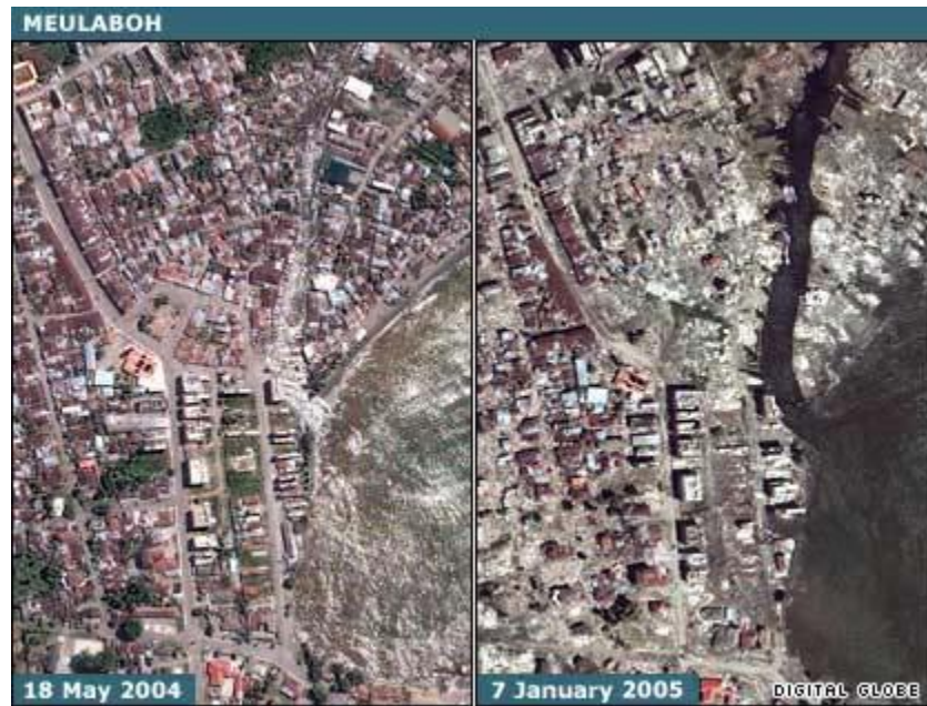
Figure 9. Aerial view of the tsunami's damage at Meulaboh, Indonesia (DigitalGlobe 2010)
