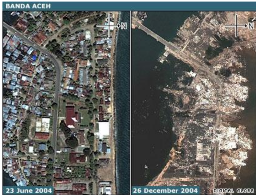
Figure 8. Aerial view of the tsunami's damage at Banda Aceh, Indonesia (DigitalGlobe 2010)
