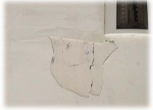
Figure 6. Filling wall cracks--3
