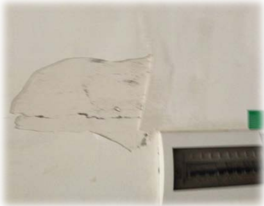
Figure 4. Filling wall cracks--1
