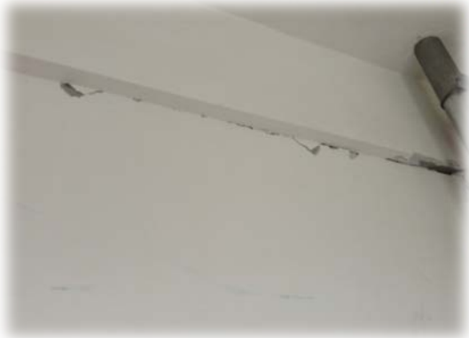
Figure 5. Filling wall cracks--2
