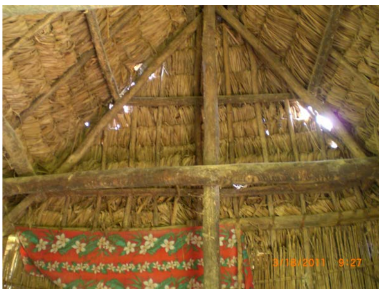
Figure 11. The kingpost ( bou ) of the house.
