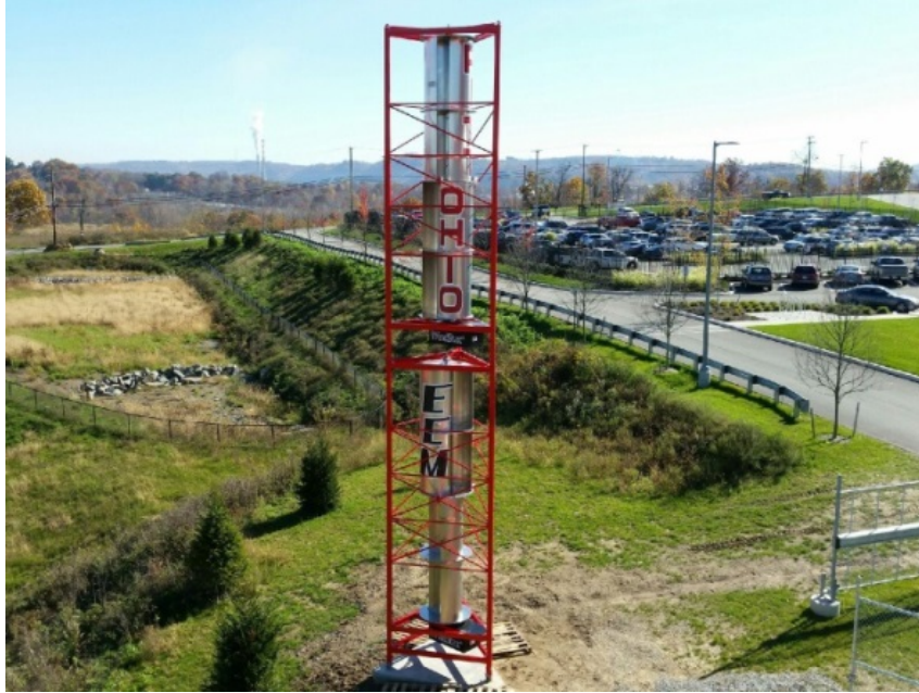
Figure 6. 5kW WindStax Vertical Axis Wind Turbine Installation
