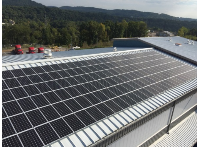
Figure 7. 50kW Photovoltaic System Installation
