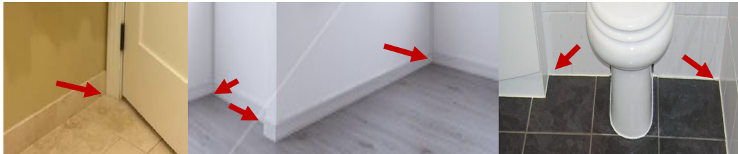
Figure 8: Tube 1- corners of the room floor and toilet floor
