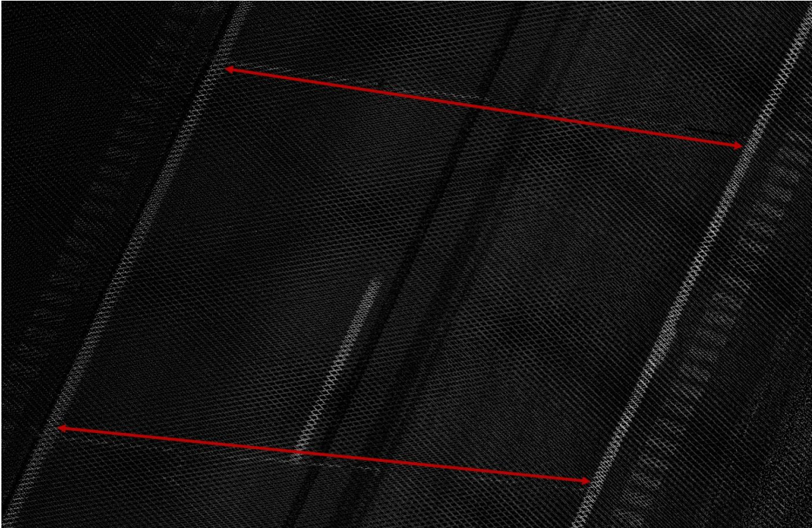
Figure D5 – Snapshot of the roadway surface as it appears in the LiDAR point cloud. The arrows indicate the approximate location of the transverse joints
