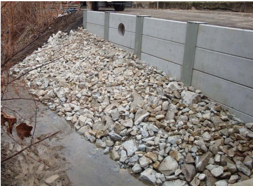
Figure 8. A soldier beam and lagging wall supports a roadway and several buried water mains along a stream in Sewickley, Pennsylvania, constructed via the top-down method.
