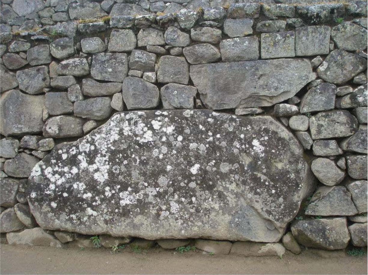
Figure 30. Wall 3 (Photo property of L.E. Vallejo)
