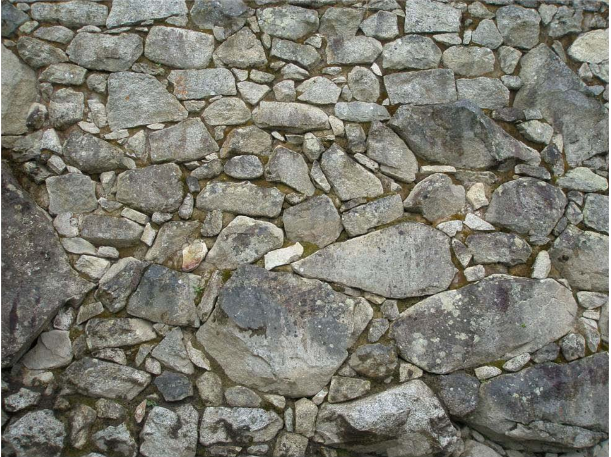
Figure 31. Wall 4 (Photo property of L.E. Vallejo)
