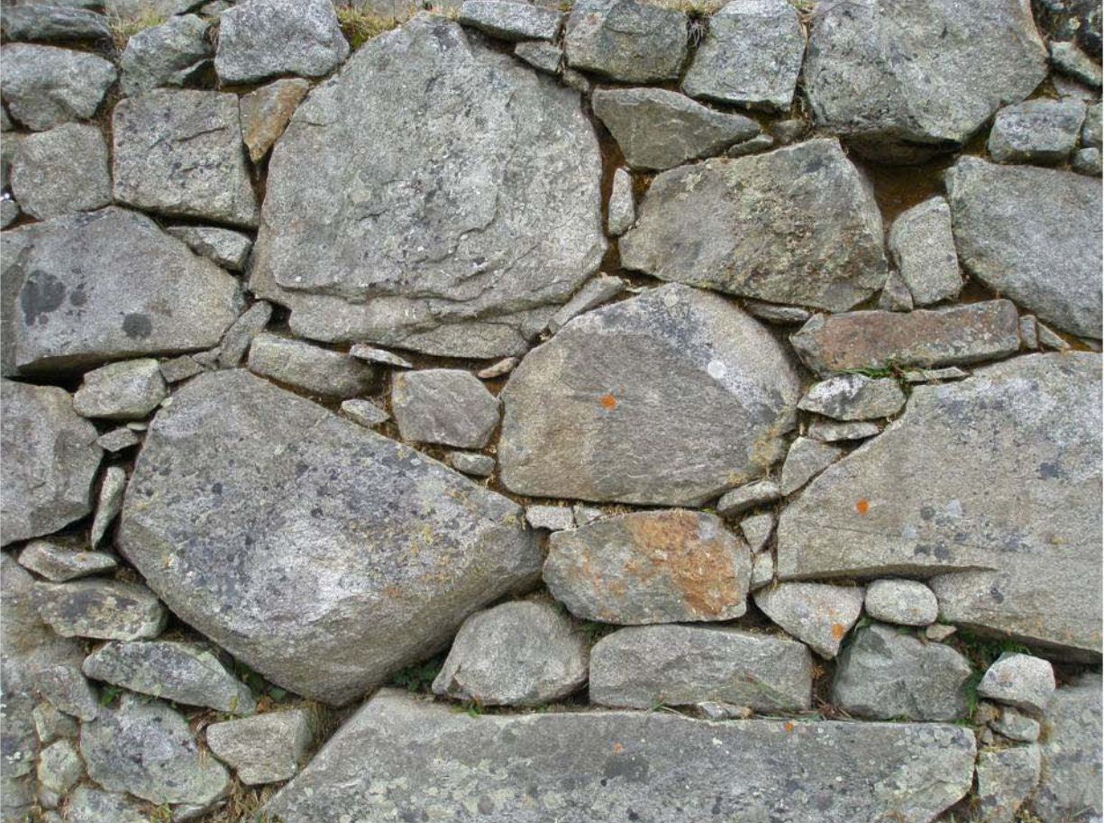
Figure 29. Wall 2 (Photo property of L.E. Vallejo)
