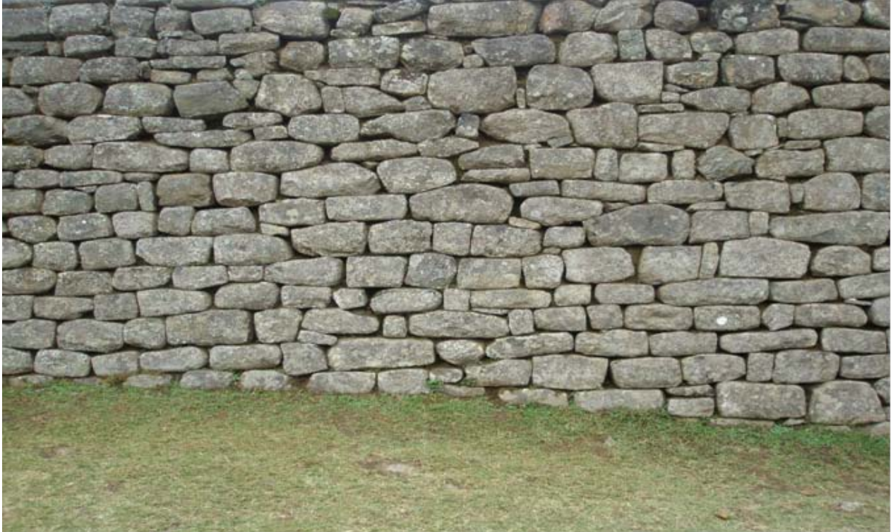
Figure 32. Wall 5 (Photo property of L.E. Vallejo)
