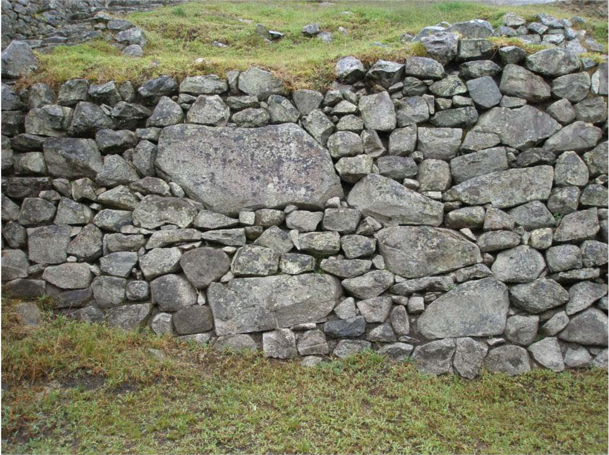
Figure 28. Wall 1 (Photo property of L.E. Vallejo)
