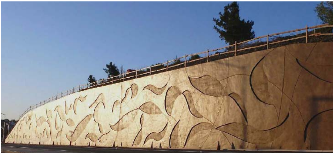
Figure 5. An example of a decorative concrete finish on a wall. (Photo property of Boulderscape, Inc., and Soil Nail Launcher, Inc.)
