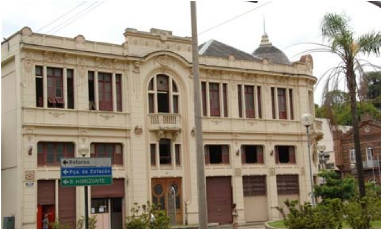
Figure 8: Municipal building where city organizations are housed. Photo Credit: Penelope Morrison
