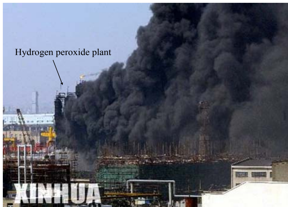
Figure 5 Explosion of a H_2O_2 plant caused by the decomposition of H_2O_2
