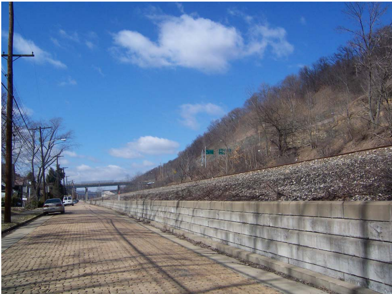
Figure 15. Glenfield and its neighbors the railroad line and Route 65.
