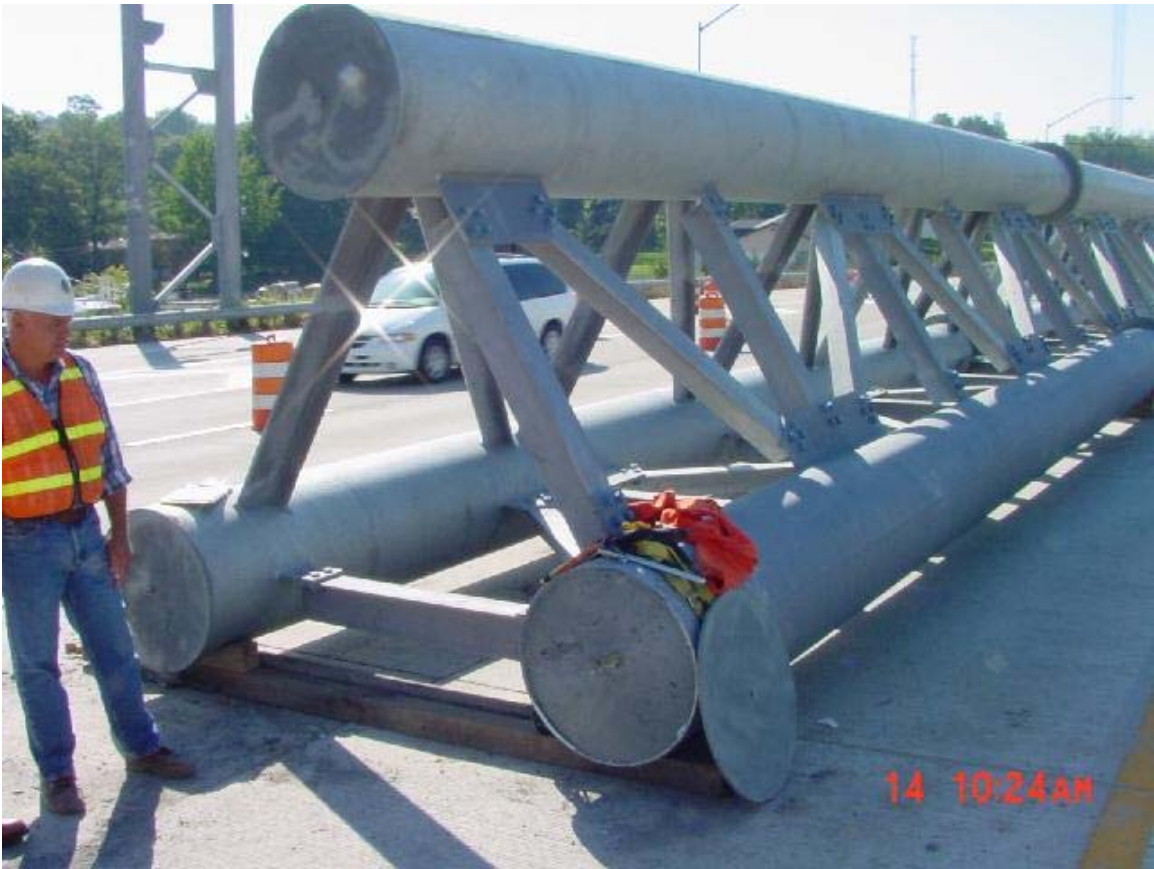
Figure 1-1: Overhead Highway Sign Truss
